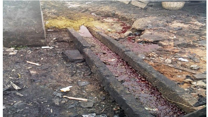
Figure 1: Manure mixed with blood flowing into open drainage from the main slaughterhouse
